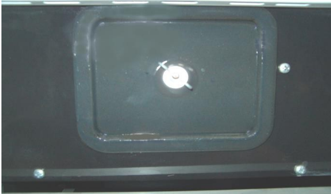
Figure 13. Inner cleaning-opening cover behind its protective cover.
